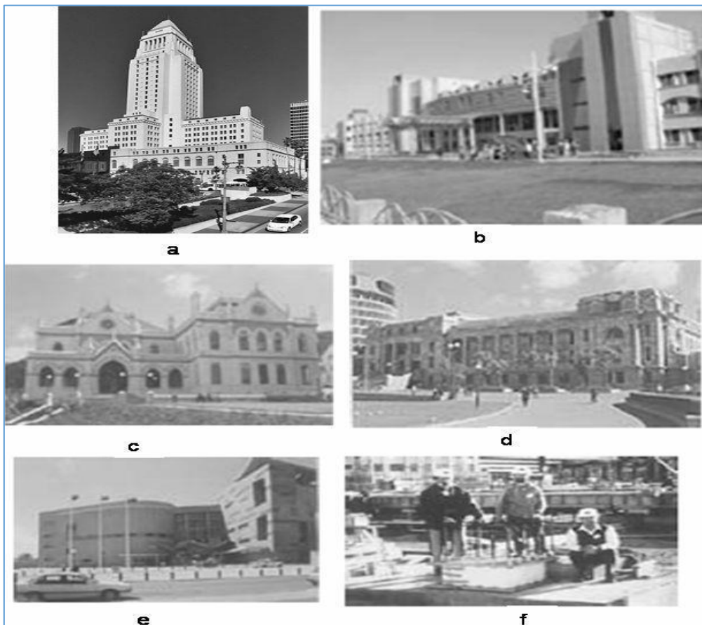
Figure 3. Some Renowned Base-isolated Structures, (a) Los Angeles City Hall, USA, (b) Bhuj Hospital, Gujrat, India, (c) New Zealand Assembly Library, (d) New Zealand Parliament, (e) Te Papa Museum of New Zealand, (f) Te Papa during Incorporation of Isolator.
